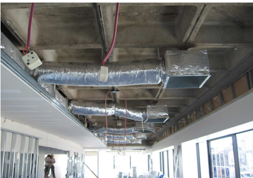
OPEN SPACE - AIR CONDITIONED FLEX DUCTS - LAYOUT MODIFICATIONS
