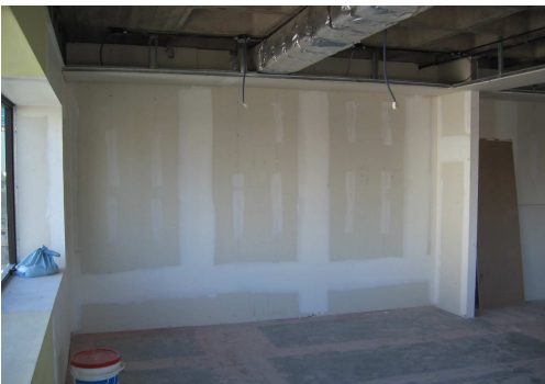
MEETING ROOM FROM INSIDE - GYPSUM BOARDS + ACRYLIC PUTTY
