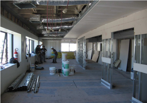
OPEN SPACE - VIEW OF CURVED WALL - METAL STRUCTURE
