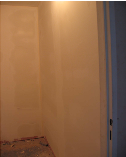
DATA CENTER FROM INSIDE - DRY WALLS - METAL STRUCTURE + RED GYPSUM BOARDS (FIRE RESISTANT) + ACRYLIC WALL PUTTY BEFORE APPLICATION OF FINISHING PAINT
