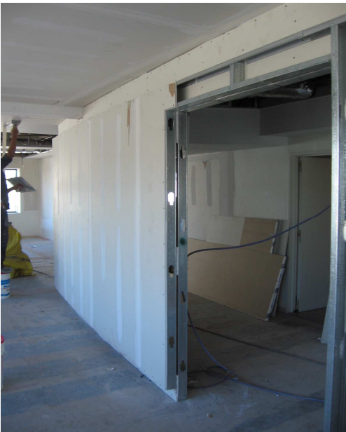
OPEN SPACE - VIEW OF CURVED WALL - DOUBLE METAL STRUCTURE + GYPSUM BOARD + ACRYLIC PUTTY
