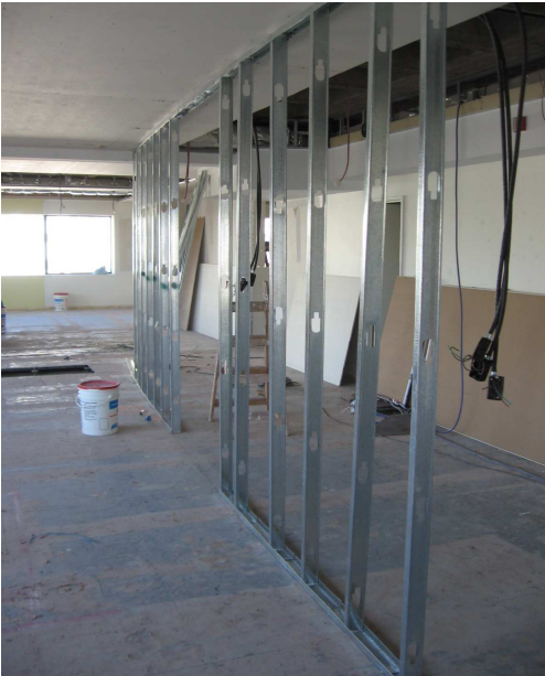
OPEN SPACE - VIEW OF CURVED WALL - METAL STRUCTURE
