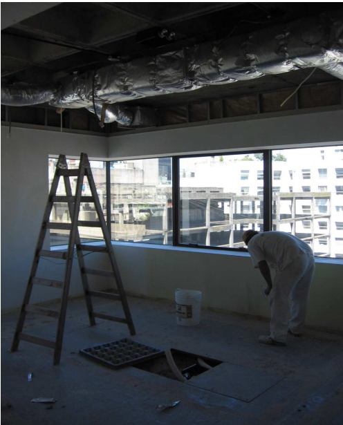
MEETING ROOM - ACRYLIC PUTTY APPLICATION BEFORE FINISHING PAINT - AIR CONDITIONED FLEX DUCTS MODIFICATIONS
