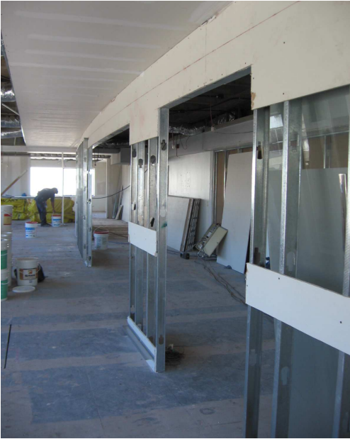
OPEN SPACE - VIEW OF CURVED WALL - METAL STRUCTURE + GYPSUM BOARD
