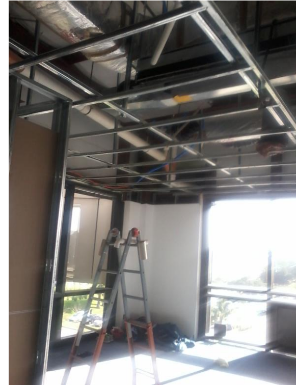
Ceiling structure laid
