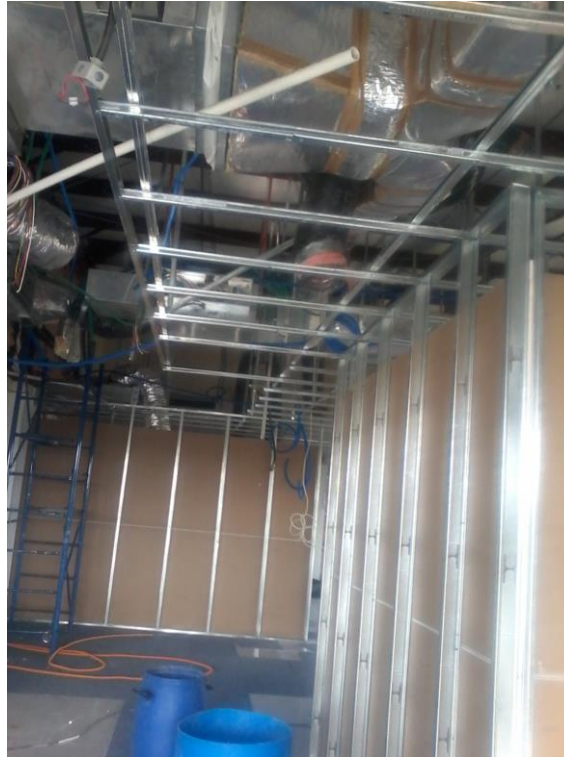
Ceiling structure laid
